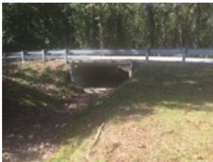
New Bridge Installation
