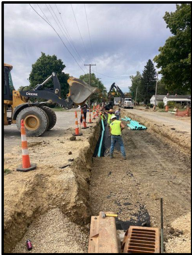
Sanitary sewer line extensions
